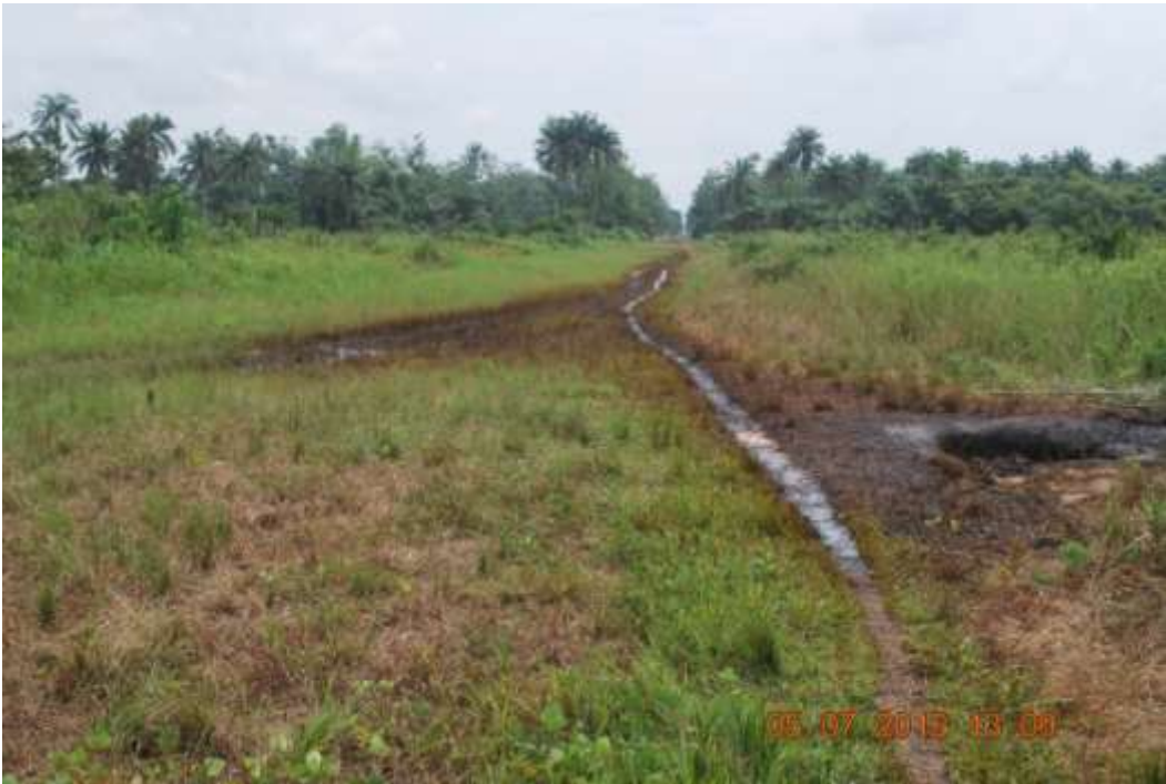
Overview: Part of spill impact on 16" Uzere-Eriemu trunkline right of way at Iyede. Picture was taken during Joint Investigation of 5 th July 2012.
