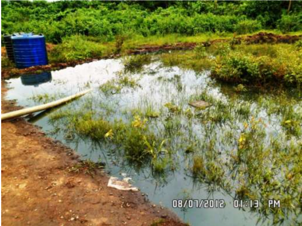
Overview: Part of spill impact on 36" Rumuekpe-Nkpoku Trans Niger Pipeline right of way at Mgbodo-Aluu.
