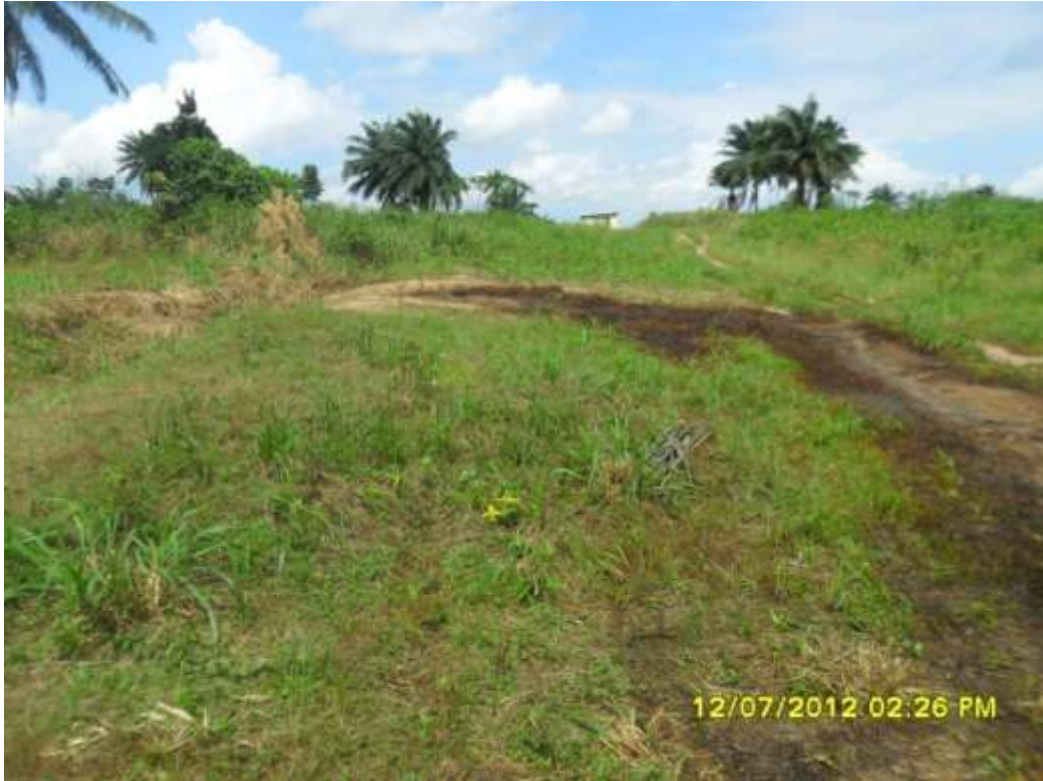
Overview: Part of spill impact on 28" Nkpoku-Bomu pipeline right of way at Gio. Picture was taken during Joint Investigation of 12 th July 2012.
