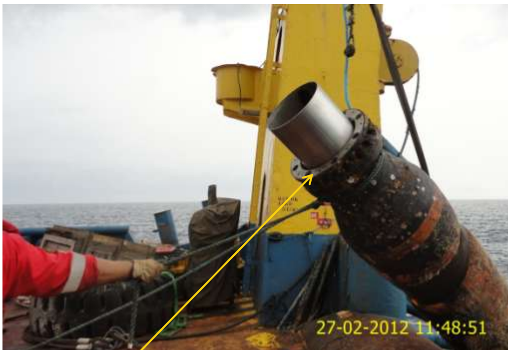
Close-up: Failed hose from SPM3 Bonny Crude Loading Platform. Picture was taken during lifting of string from sea bed on 27 th February 2012.
