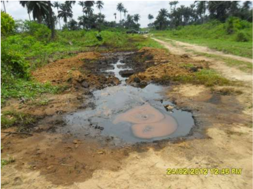
Overview: Part of spill impact on 6" Obigbo north – Ogale pipeline right of way at KomKom. Picture was taken during Joint Investigation of 24 th February 2012.
