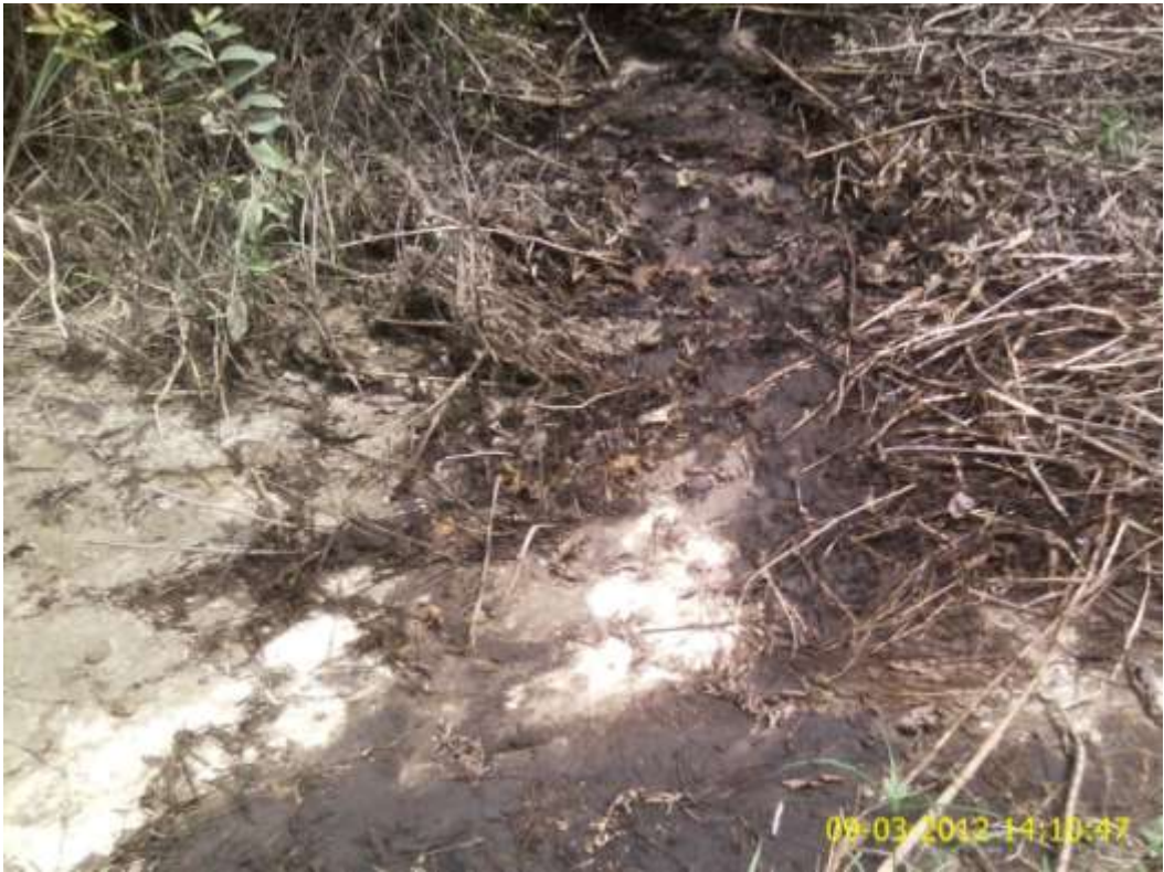
Overview: Part of spill impact on 12" Adibawa-Okordia pipeline right of way at Edagberi-Betterland. Picture was taken during Joint Investigation of 9 th March 2012.
