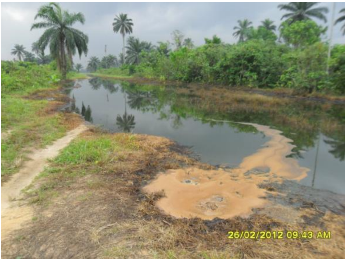
Overview: Part of spill impact at 28" Nkpoku – Bomu Pipeline route in Aleto-Nchia-Eleme. Picture was taken during Joint Investigation of 26 February 2012.
