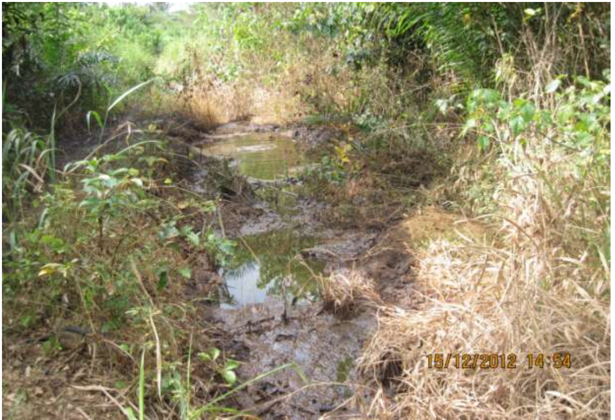
Overview: Part of spill impact on 4 inch Otamiri Well 8L Flowline at Umuechem. Picture was taken during Joint Investigation of 15 th Dec. 2012.
