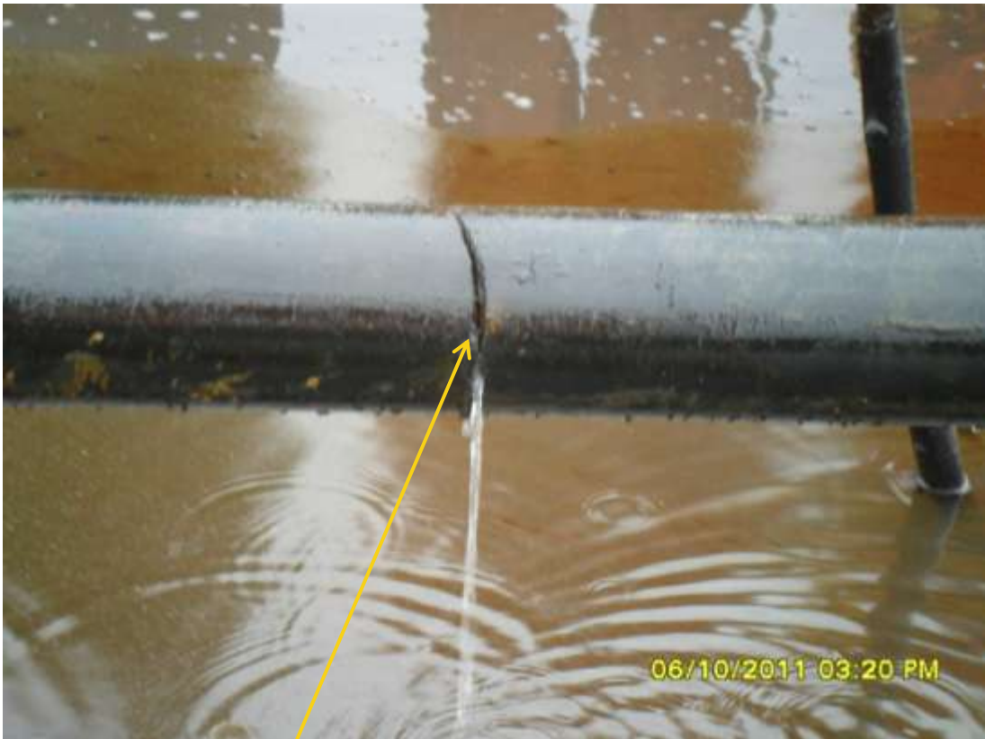
Close-up: Hacksaw cut on Cawthorne Channel III Well43S flowline right of way at Moneykiri. Picture taken during Joint Investigation of 6 th October, 2011.
