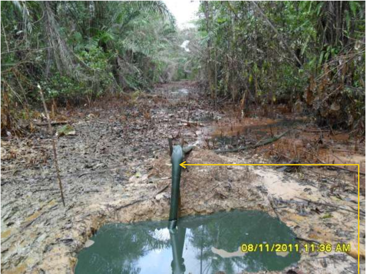
Overview: Part of spill impact on 10" Diebu Creek pipeline at Oporoma right of way. Hose used for bunkering can be seen in the photo.
