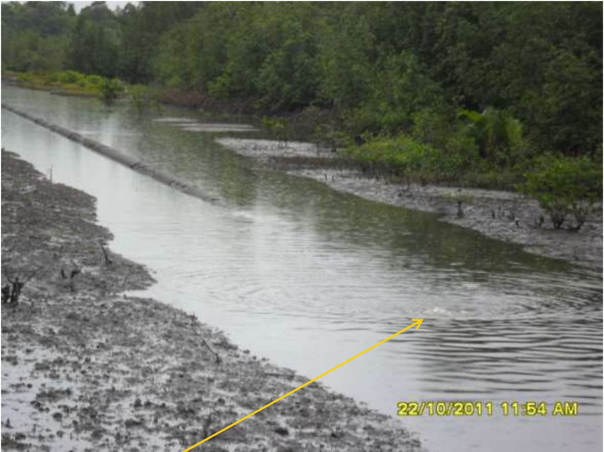
Overview: Bubbling observed on 20" Buguma-Alakiri pipeline right of way at Bakana. Picture was taken during Joint Investigation of 22 nd October, 2011.
