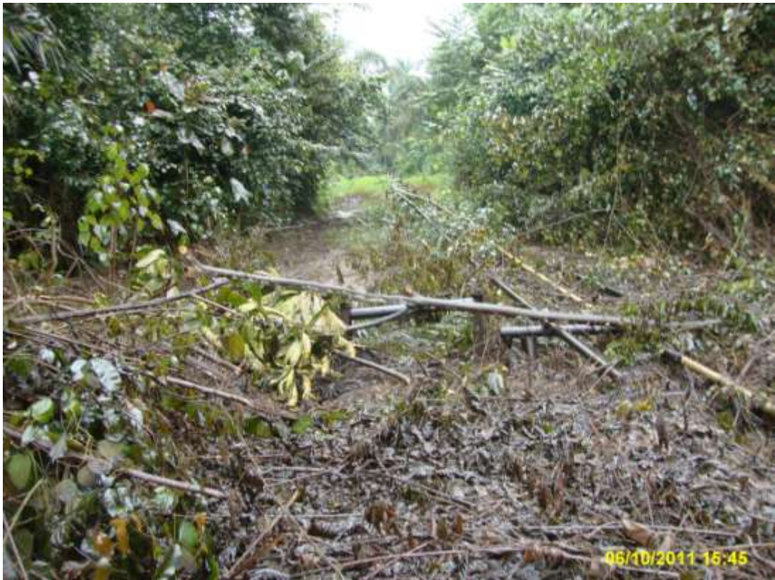
Overview: Part of spill impact on 4" ImoRiver1 Well30S flowline right of way at Igiriukwu. Picture taken during Joint Investigation of 6 th October, 2011.
