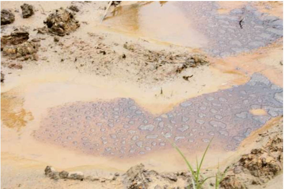
Overview: Part of spill impact at 24" Trans Ramos pipeline right of way at Aghoro. Picture was taken during Joint Investigation of 3 rd November, 2011.
