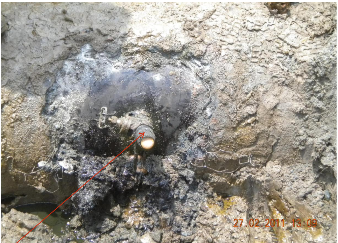
Close-up: Spill due to illegally welded points on 28" Bomu- Bonny Pipeline at Bodo West.. Picture taken during Joint Investigation of 27 th February, 2011.
