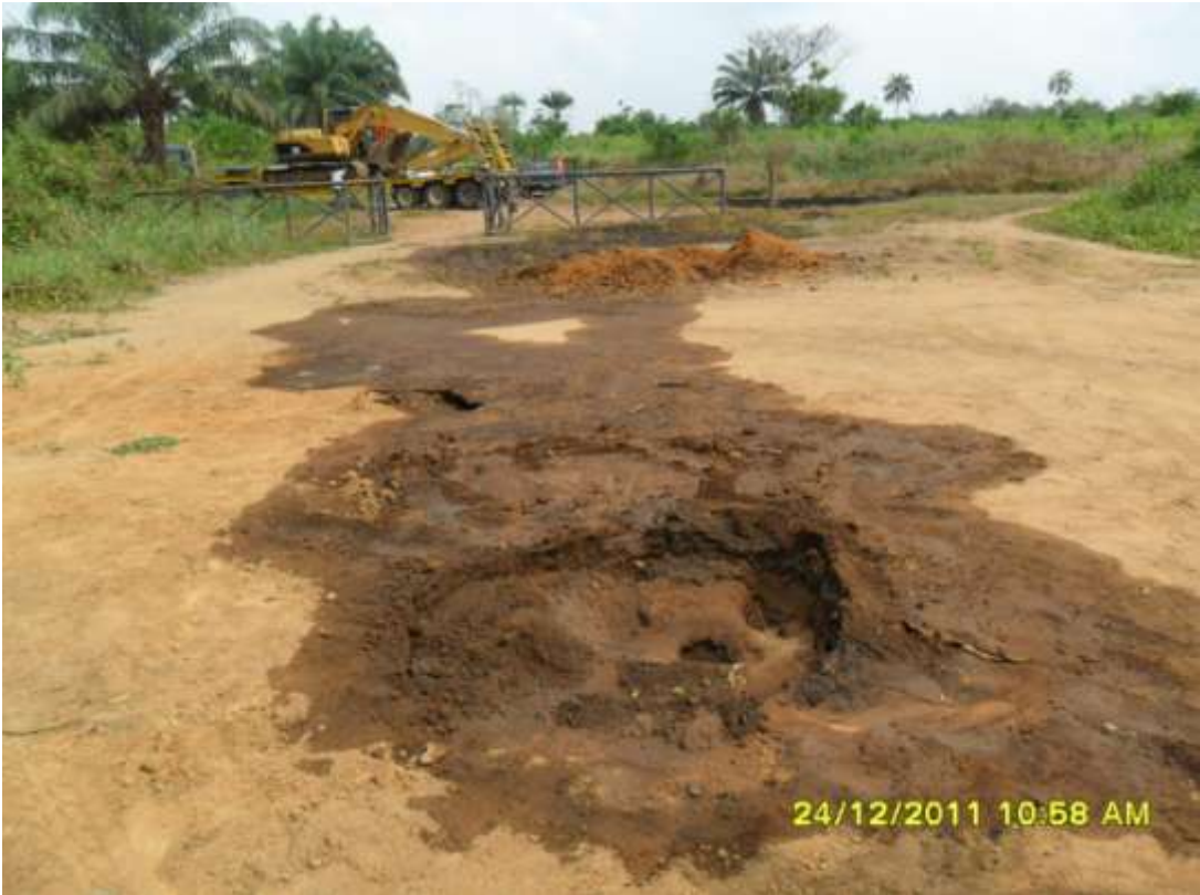
Overview: Part of spill impact on 18" Assa-Rumuekpe pipeline right of way at Awara. Picture was taken during Joint Investigation of 24 th December 2011.
