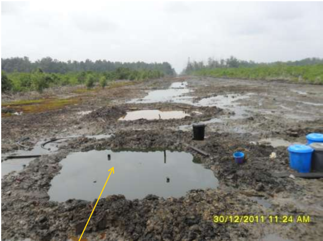
Overview: Location of illegal fittings on 24" Nembe Creek pipeline right of way at Nembe Bassambiri. Picture was taken during Joint Investigation of 30 th December 2011.
