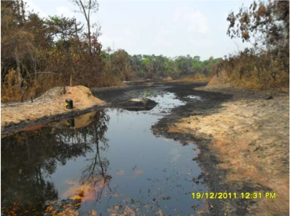
Overview: Part of spill impact on 16" NunRiver-Kolocreek pipeline right of way at Aguobiri. Picture was taken during Joint Investigation of 19 th December, 2011.
