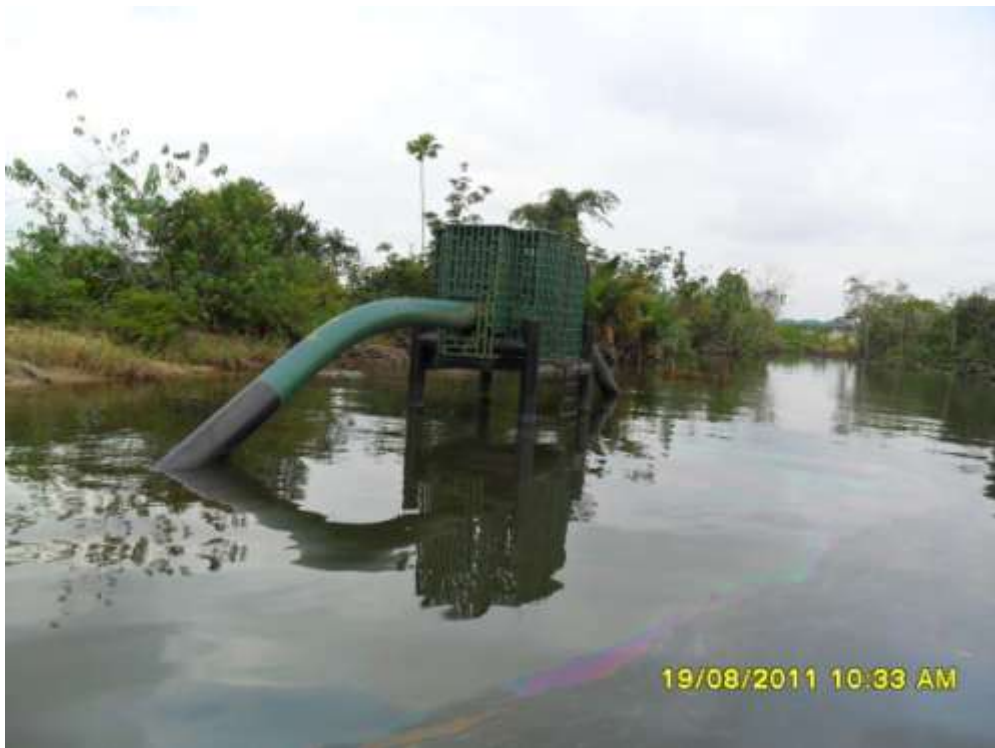
Overview: Part of spill impact on Buguma-Alakiri trunkline right of way at Abiama. Picture taken during Joint Investigation of 19 th August, 2011.
