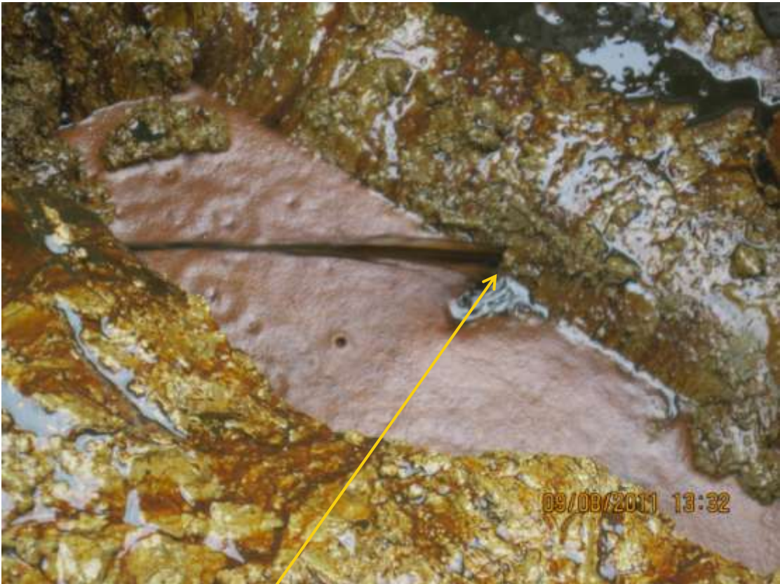
Close-up: Spill due to hacksaw cut on 14in Okordia-Rumuekpe pipeline at Ikarama. Picture taken during Joint Investigation of 9 th August, 2011.
