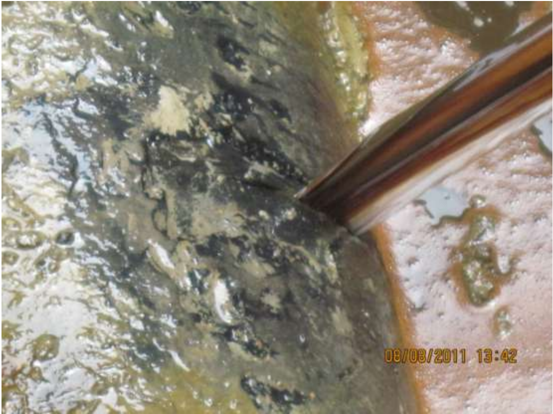
Close-up: Spill due to hacksaw cut on Adibawa-Okordia pipeline at Ikarama. Picture taken during Joint Investigation of 8 th August, 2011
