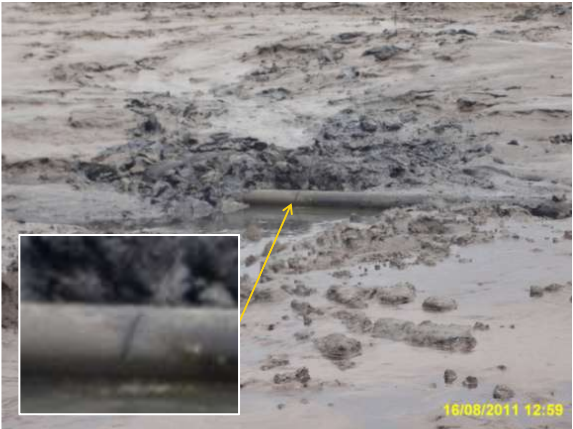
Close-up: Spill due to hacksaw cut on Akaso Well 10L flowline at Cawthorne Channel. Picture taken during Joint Investigation of 16 th August, 2011.
