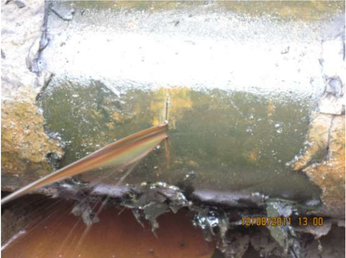
Close-up: Spill due to hacksaw cut on 14" Okordia-Rumuekpe pipeline at Ikarama. Picture taken during Joint Investigation of 12 th August, 2011.
