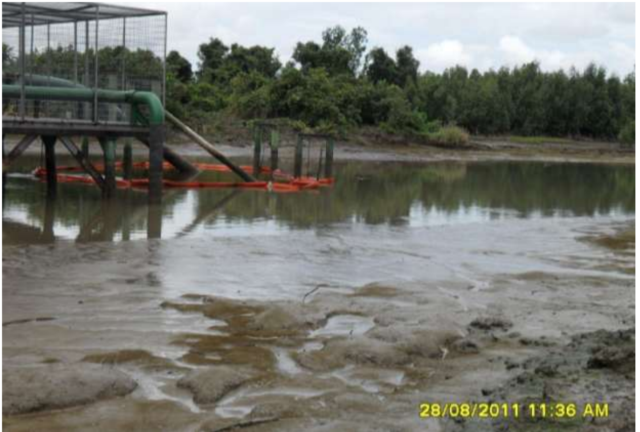
Overview: Part of the spill impact on 10" Ekulama-Sanbarth pipeline at Sanbarth. Picture taken during Joint Investigation of 28 th August 2011
