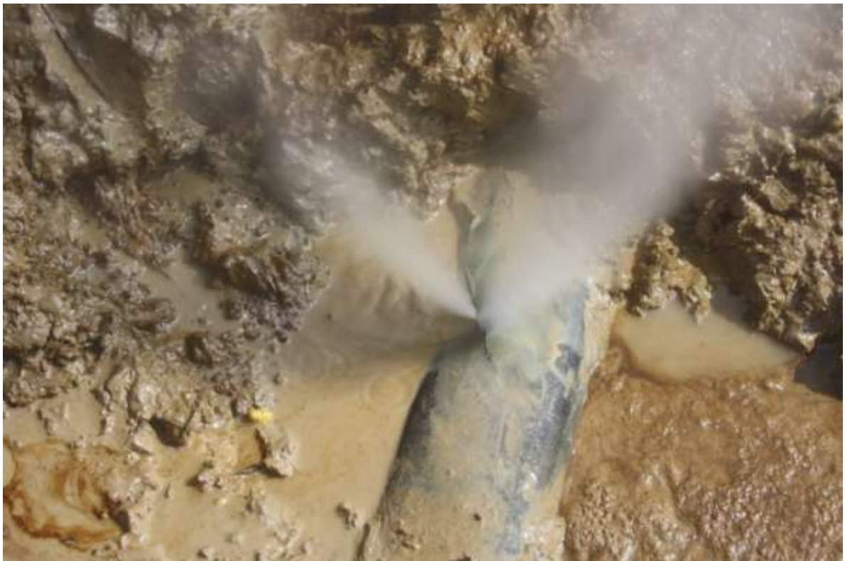
Close-up: Spill due to damage by 3 rd party equipment on 6" Utorogu-Ughelli West gasoline at Iwhrekan. Picture taken during Joint Investigation of 25 th August, 2011.
