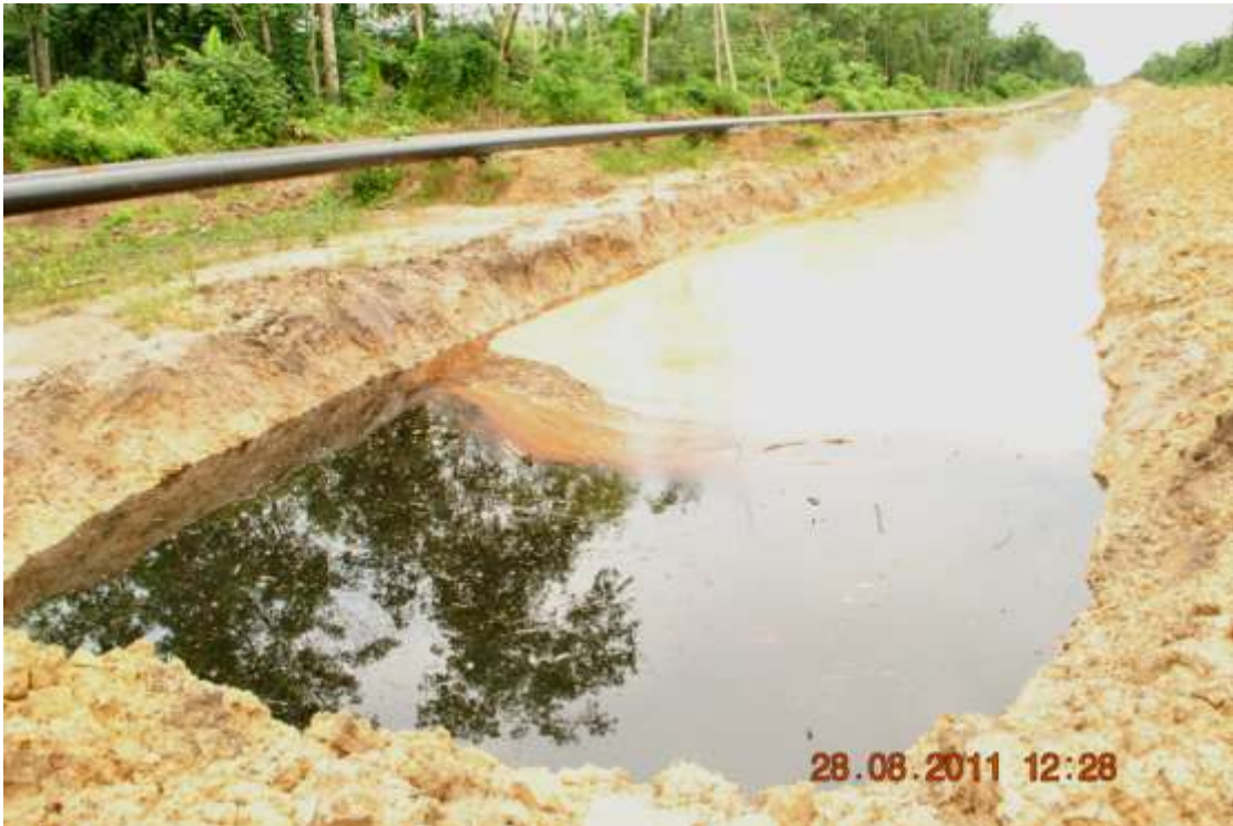
Overview: Part of spill impact on 10" Utorogu-UPS right of way at Ughevwighe. Picture taken during Joint Investigation of 28 th August, 2011.
