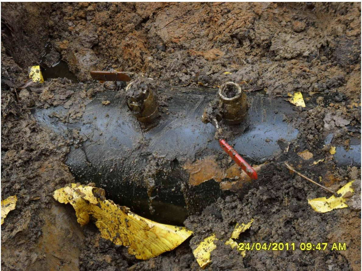
Close-up: Illegally welded points on 12" Imo 2 – Ogale Pipeline at Owaza. Picture was taken during JIV of 24 April 2011
