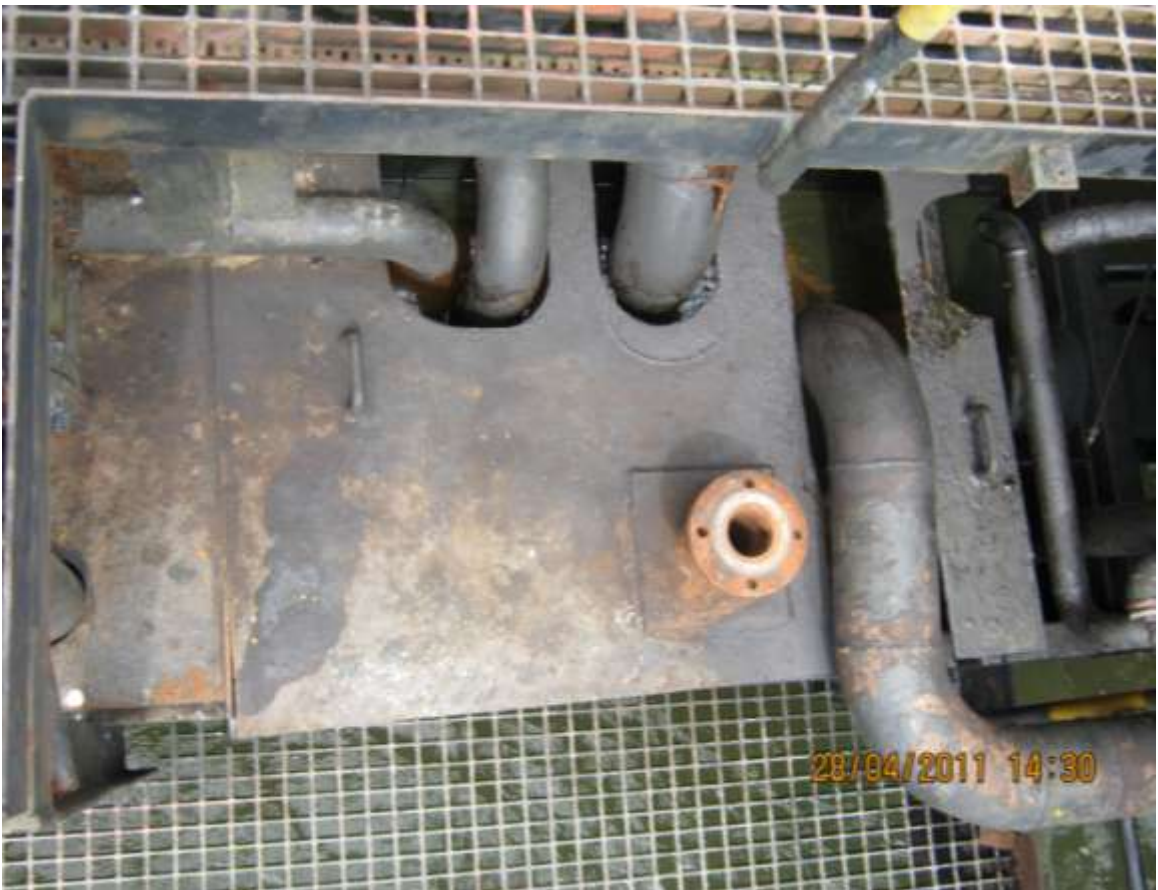
Close-up: Saver-pit source of over flow at Nembe creek 2 flow station in Nembe . Picture was taken during JIV of 28 th April, 2011
