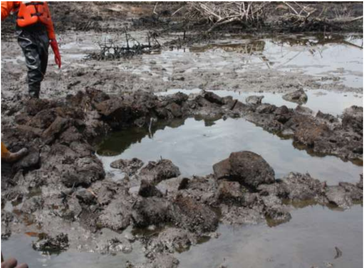
Overview: Extent of the spill incident impact on 24" UPS-Rapele trunkline at Ugbokodo. Picture taken during JIV of 6 th April, 2011
