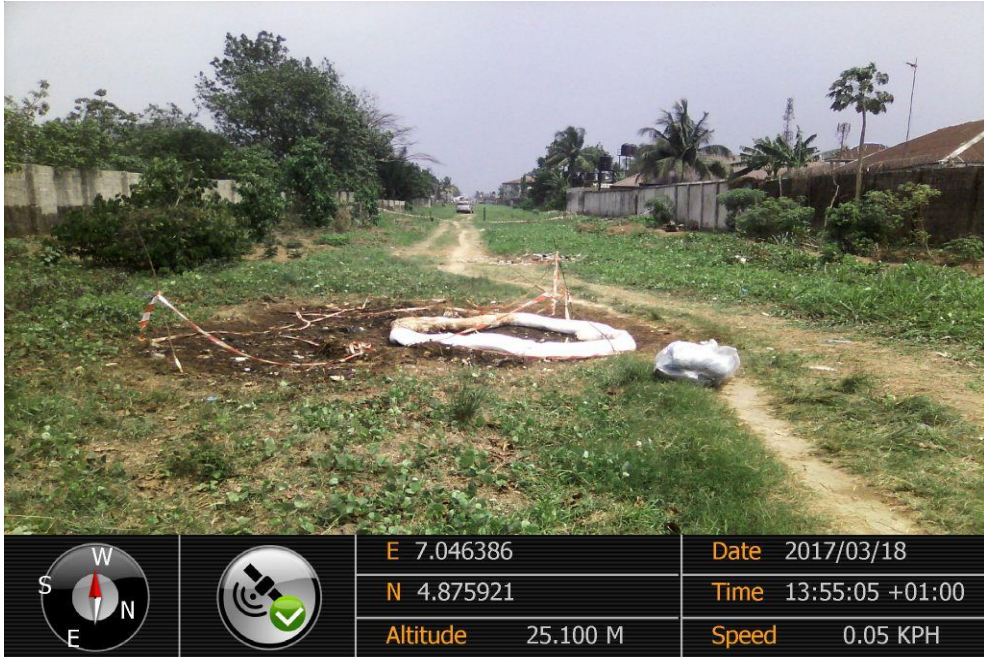
Overview: Part of spill impact on 28" Nkpoku-Bomu Pipeline at Elimgbu. Picture was taken during Joint Investigation of 18 th March 2017.
