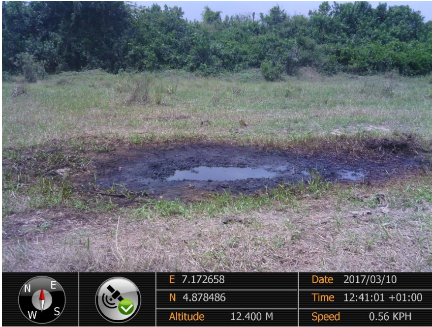
Overview: Part of spill impact on 12" Imo River-Ogale Pipeline at Komkom. Picture was taken during Joint Investigation of 10 th March 2017.
