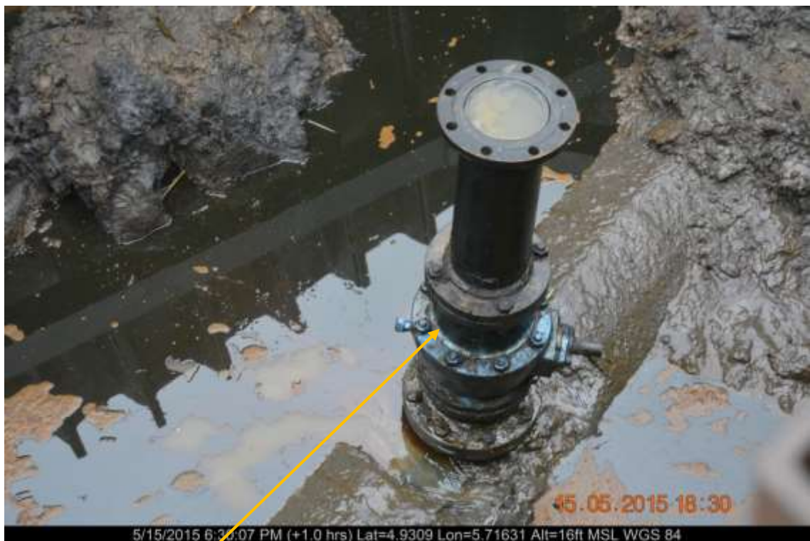
Close-up: Illegal fitting on 20" Opukushi – Brass Creek Pipeline at Tamogbene. Picture was taken during Joint Investigation of 15 th May 2015.
