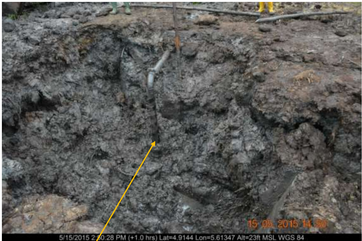
Close-up: Illegal fitting on 16" Tunu – Brass Creek Pipeline at Agbidiana. Picture was taken during Joint Investigation of 15 th May 2015.
