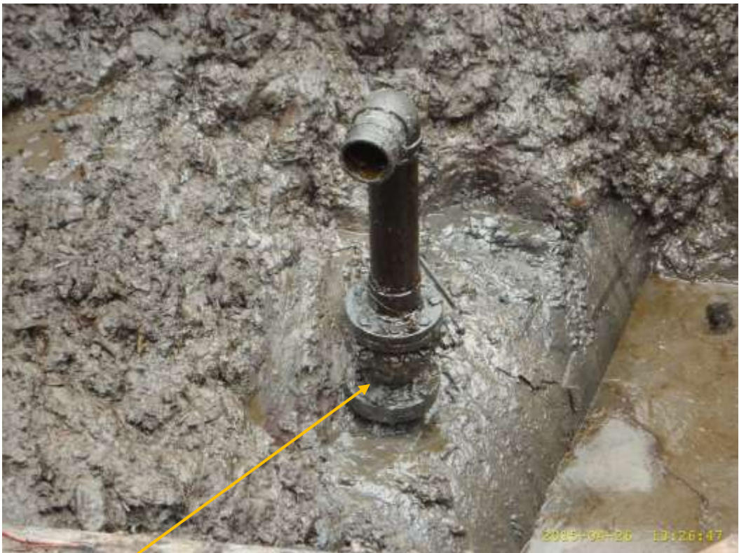
Close-up: Illegal fitting on 28" Bomu-Bony Trans Niger Pipeline at Bodo West. Picture was taken during Joint Investigation of 26 th April 2015.
