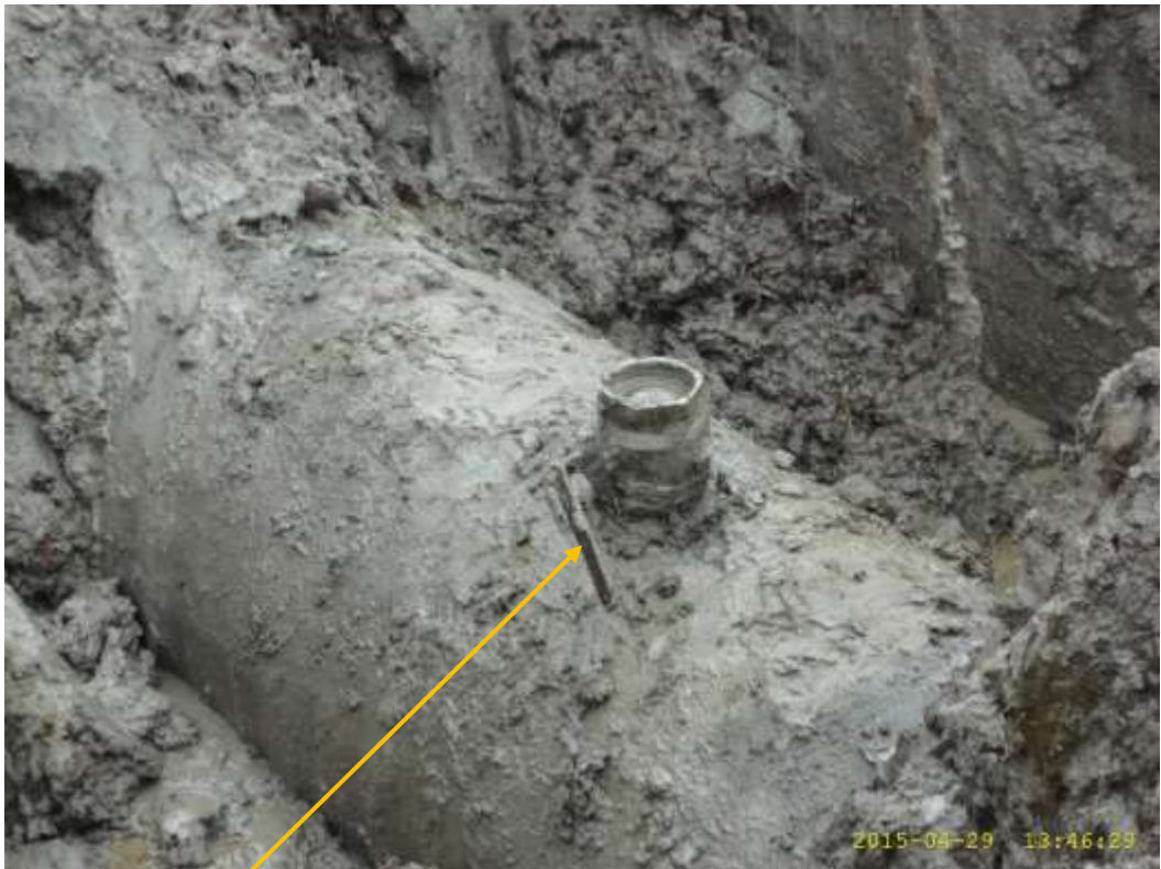
Close-up: Illegal fitting on 28" Bomu-Bonny Trans Niger Pipeline at Bodo West. Picture was taken during Joint Investigation of 29 th April 2015.
