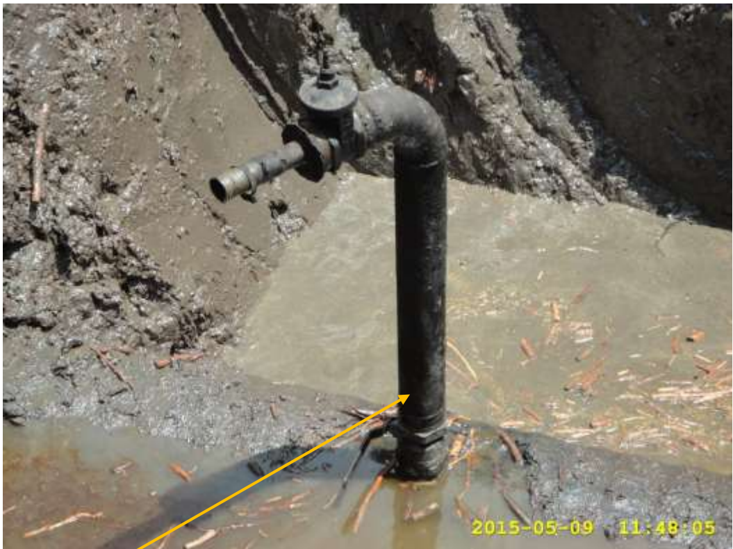
Close-up: Illegal fitting on 28" Bomu-Bonny Trans Niger Pipeline at Otokolomabie/Oloma. Picture was taken during Joint Investigation of 9 th May 2015.
