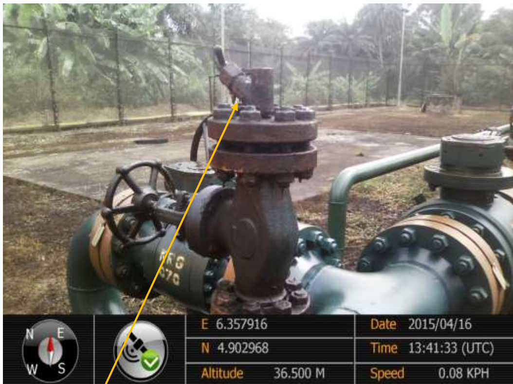
Close-up: Former Location of missing Cork Valve Gauge (1) on Kolocreek Manifold at Otusega. Picture was taken during Joint Investigation of 16 th of April 2015.
