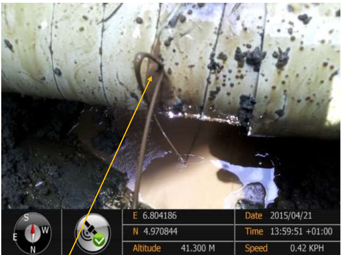
Close-up: Hacksaw cut on 4" Obele-Ibaa Pipeline at Ibaa/Omueze. Picture was taken during Joint Investigation of 21 st April 2015.
