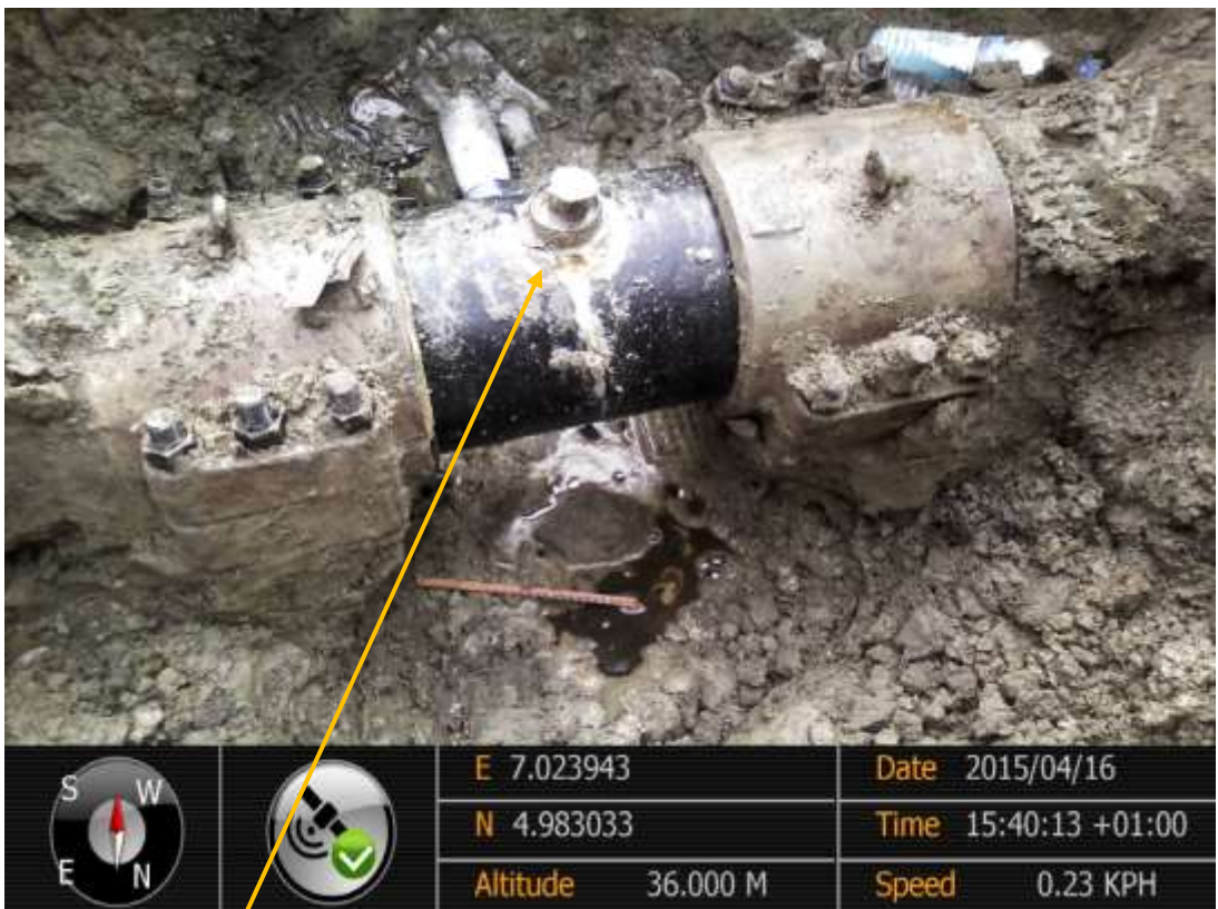
Close-up: Illegal fitting on 8" Umuechem-Nkpoku Pipeline at Omunwei. Picture was taken during Joint Investigation of 16 th April 2015.
