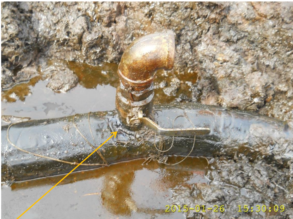
Close-up: Illegal fitting on Santa Barbara Well 14S Flowline at Nembe - Bassambiri. Picture was taken during Joint Investigation of 26th January 2015.
