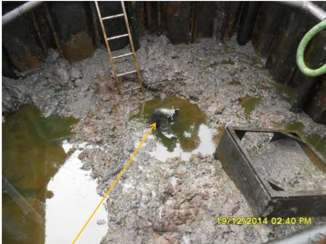
Close-up: Illegal fitting on 30" Nembe Creek Pipeline at Km45 Awoba. Picture was taken during Joint Investigation of 19 th December 2014.
