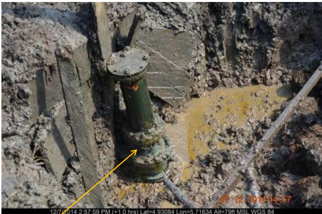
Close-up: Illegal fitting on 20" Opukushi – Brass Creek Pipeline at Amabulou. Picture was taken during Joint Investigation of 7 th December 2014.
