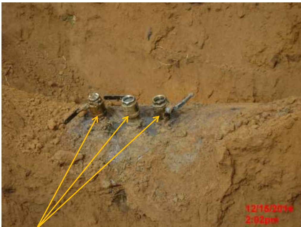
Close-up: Illegal fittings on 28" Nkpoku-Bomu Pipeline at Elenwo. Picture was taken during Joint Investigation of 15 th December 2014.
