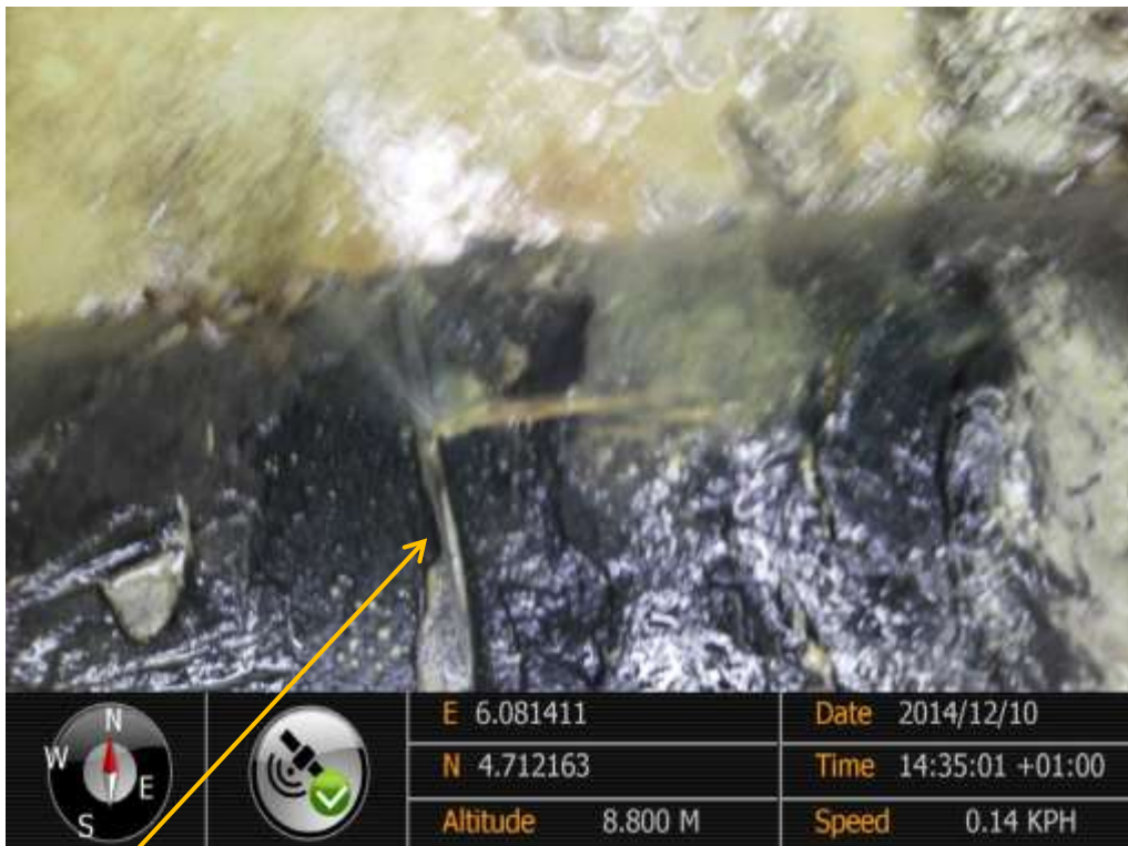
Close-up: Hacksaw cut on 10" Diebu Creek Nun River Pipeline at Ekowe. Picture was taken during Joint Investigation of 10 th December 2014.
