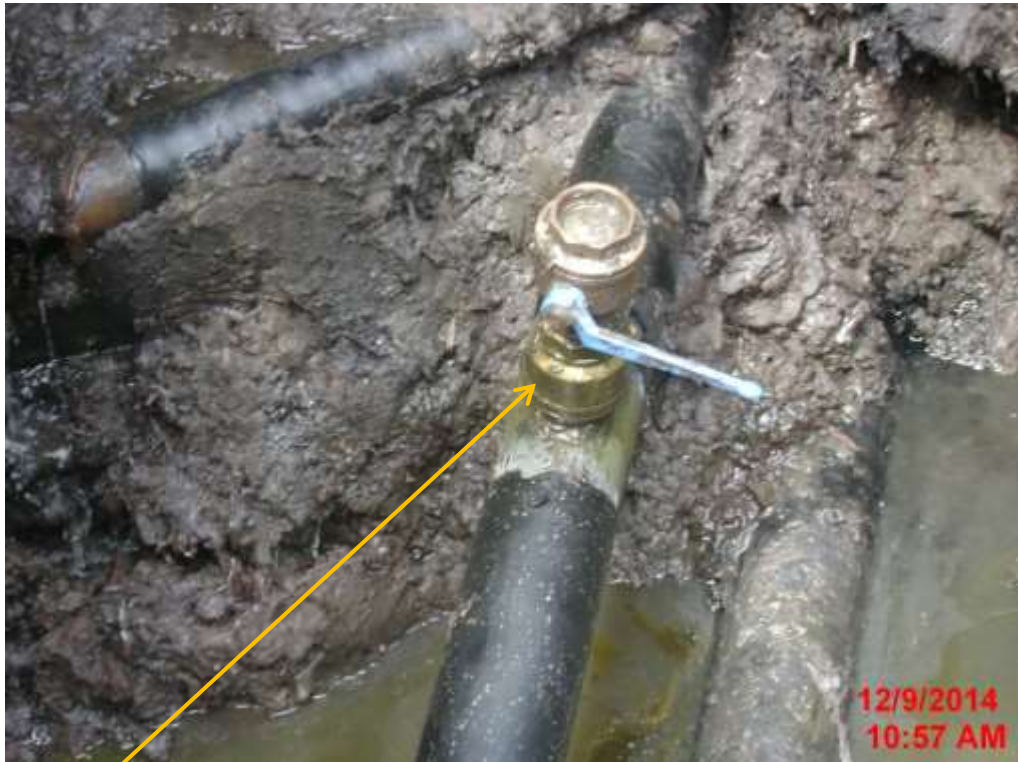
Close-up: Illegal fitting on 6" Odeama-Tora Pipeline at Nembe/Bassambiri. Picture was taken during Joint Investigation of 9 th December 2014.
