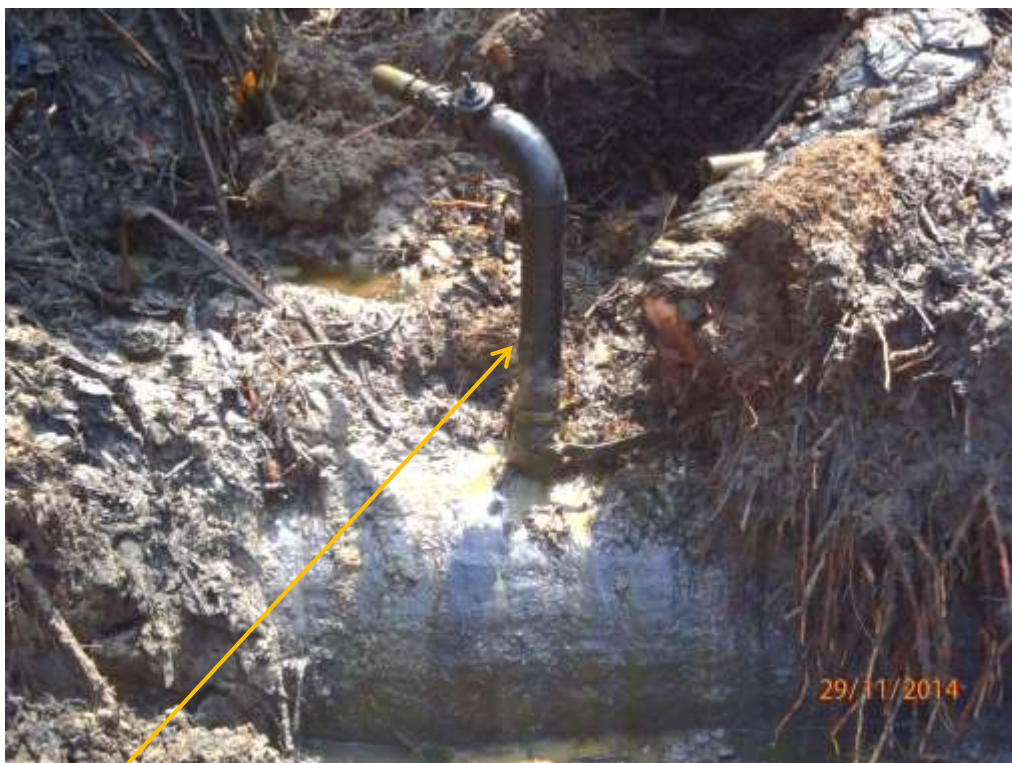
Close-up: Illegal fitting on 28" Bomu-Bonny Pipeline at Oloma. Picture was taken during Joint Investigation of 29 th November 2014.
