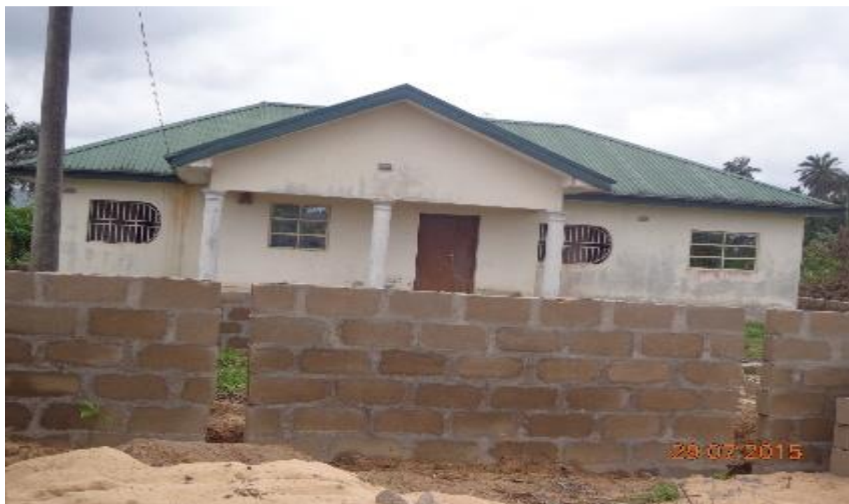
Plate 4.15b: Public Health Center at Obunagha is being constructed
