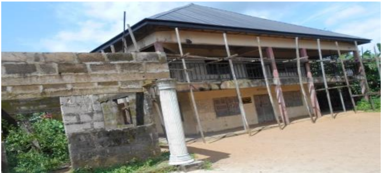
Plate 4.14g: Typical Block wall houses in the communities
