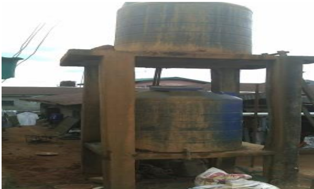
Plate 4.14 jPrivate borehole water supply in one of the communities
