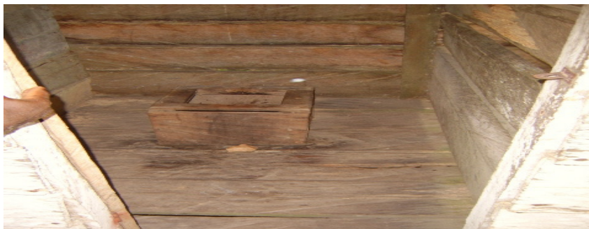
Plate 4.1c: A typical overhung toilet in Ezetu community
