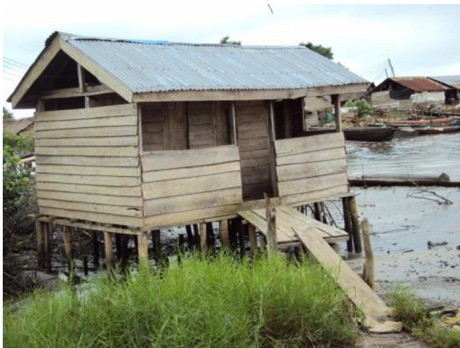
Plate 4.44: A Toilet in Newtown Community
