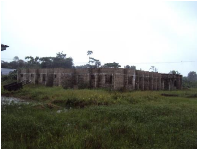
Plate 4.54: New Health Center Under Construction in Kula Community
