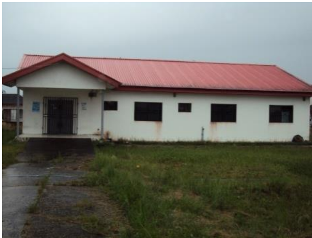
Plate 4.52: Elem Sangama Comprehensive Health Center Under Lock
