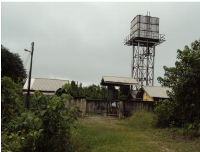
Plate 4.42: A Non-functional Water Facility at Freetown
