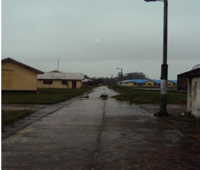
Plate 4.46: Built-Up Housing Structures at Elem Sangama
