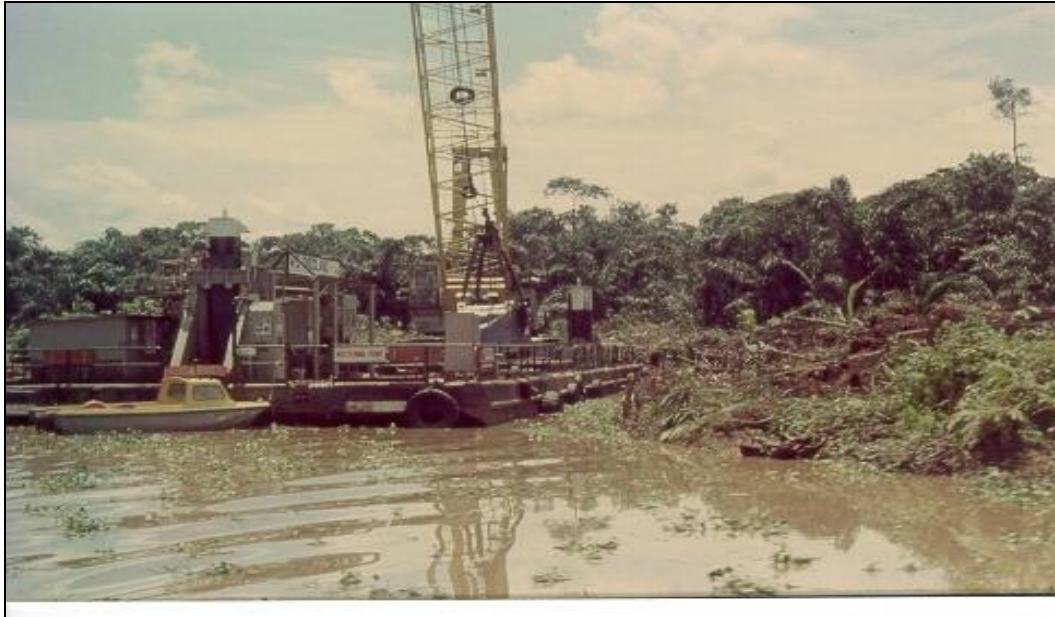
Plate 5.2: Grab dredger in action in Opukushi field.
