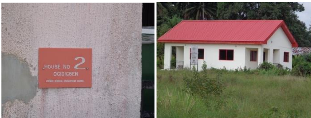
Plate 4.11.6: One of the houses built in Ogidigben by the Itsekiri Regional Development Council
