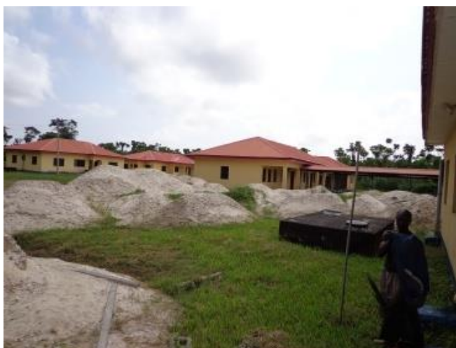
Plate 4.11.10: Cottage hospital in Ogidigben being renovated
