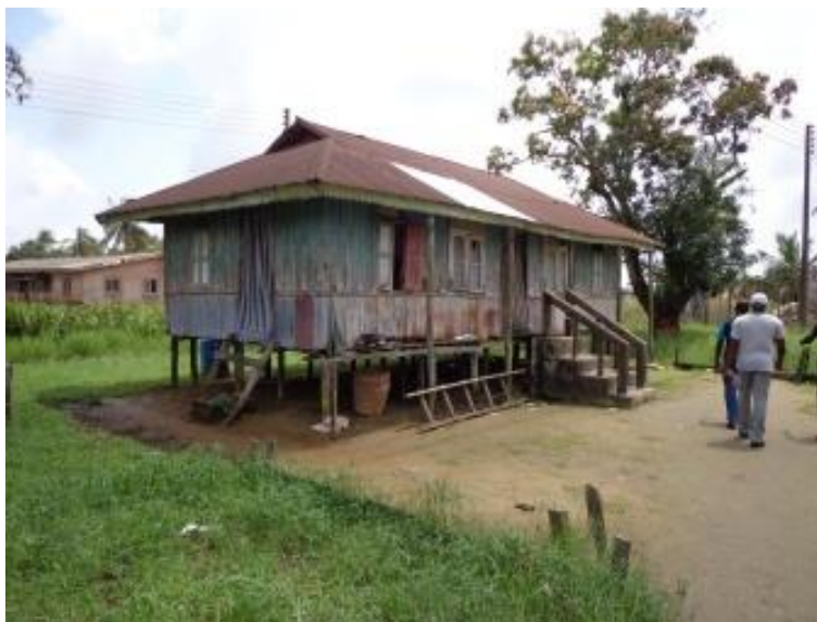
Plate 4.11.5: Raised house in a host community
