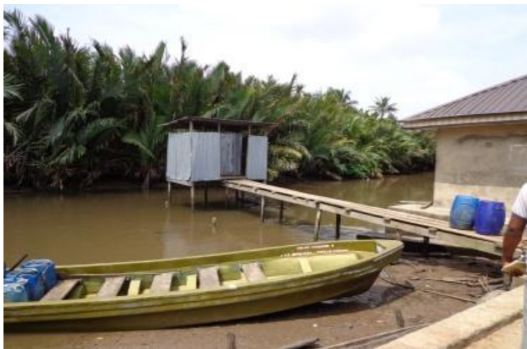
Plate 4.11.4: The jetty-type toilet is the commonest toilet in the host communities
