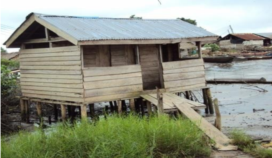
Plate 4.2.10.6: An Over-hung toilet in a Riverine Community in Bayelsa State
