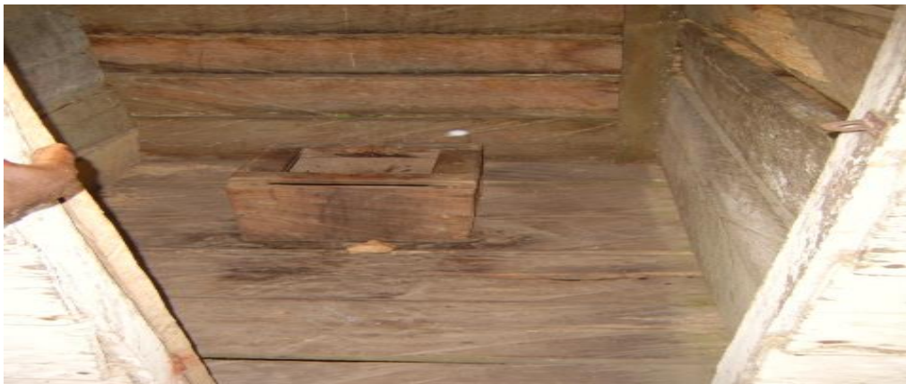
Plate 4.2.9.3: A typical overhung toilet in Ezetu community
