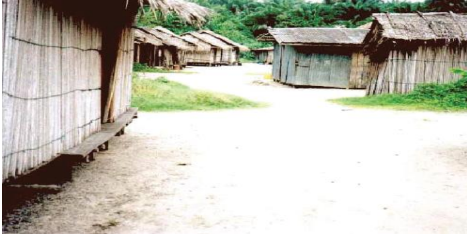
Plate 4.2.9.2: Typical Residential housing in the coastal communities
